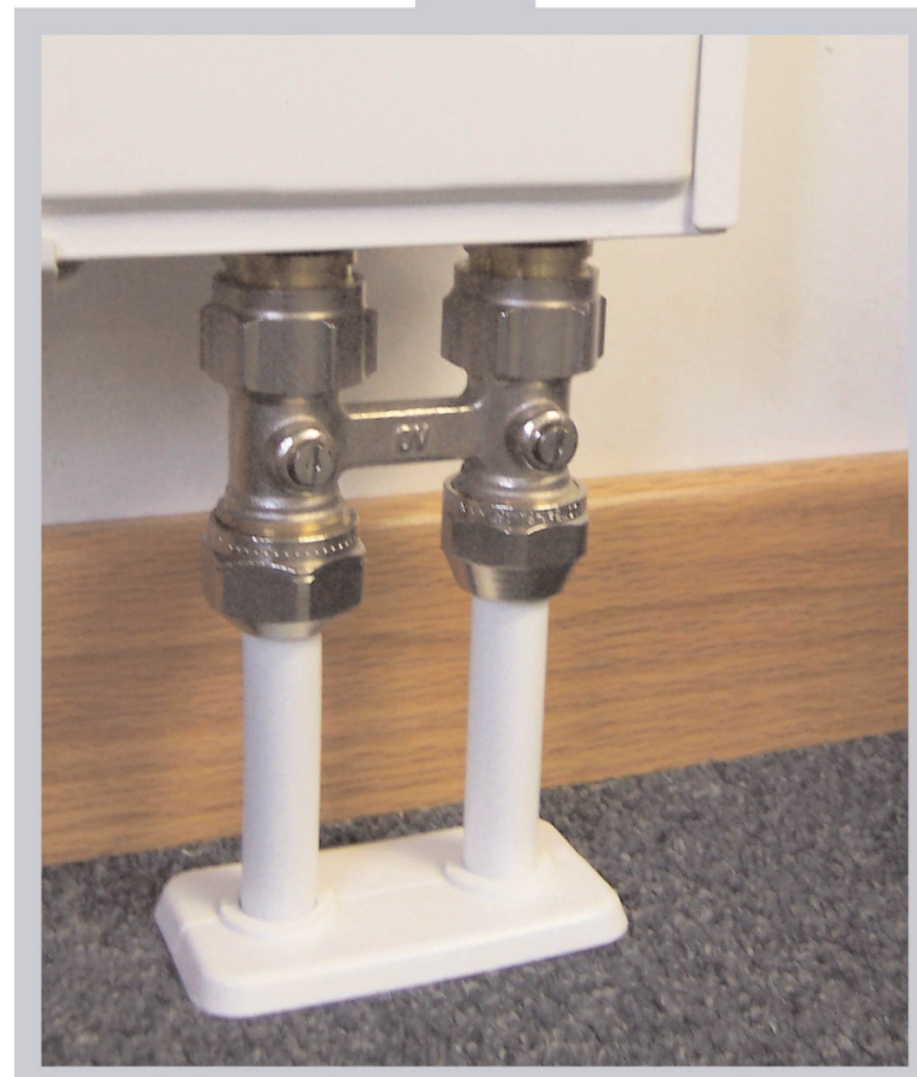
Isolation valves on supply and return piping
